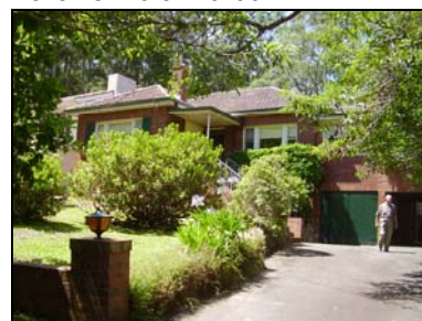
No. 23 Kimbarra Road
