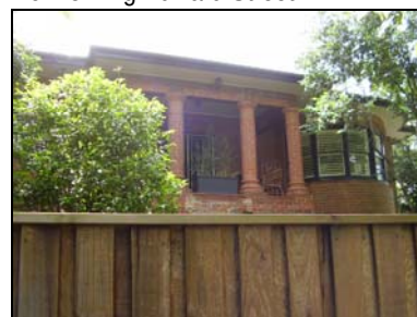
No. 35 Mona Vale Road
