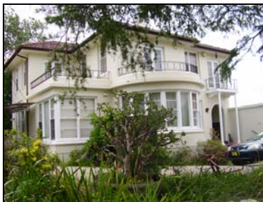
No. 85 Mona Vale Road
