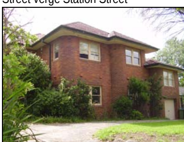
No. 81 Mona Vale Road
